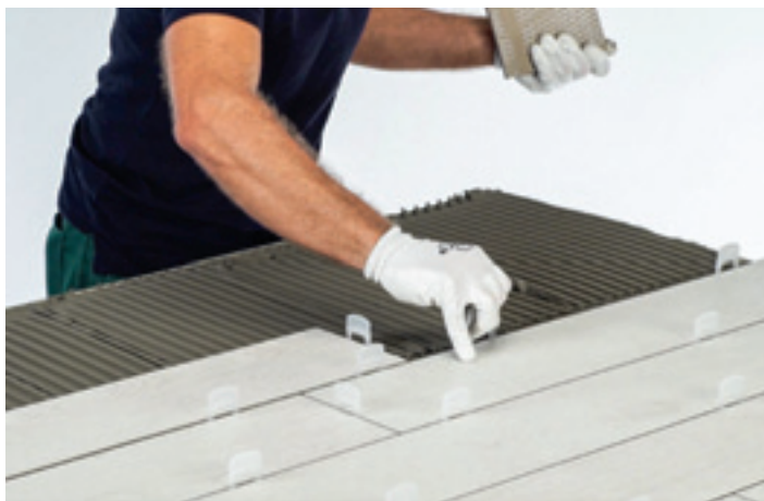
disposable clips installation
