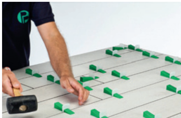
wedges and clips removal
