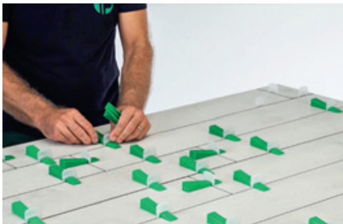
levelling wedges insertion
