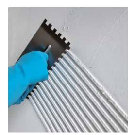
Spreading white Fix & Grout Brick diagonally with a No. 10 notched trowel
