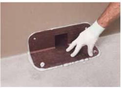
3. Place Drain Front in position and press down lightly so that it is embedded in Adesilex PG4
