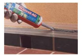
13. Seal with Mapesil AC in correspondence with the skirting board-wall fillet joint
