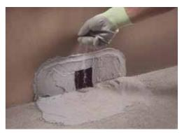
5. Smooth over with a flat trowel and, while the product is still fresh, sprinkle on a layer of 0.5 spheroid quartz to form a rough layer to help the specified MAPEI waterproofing product form a good bond
