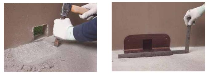
1. Make a hole in the parapet and floor large enough to insert the Drain Front. Make sure it is perfectly level with the horizontal and vertical surfaces
