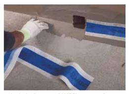
7. Apply the first coat of MAPEI waterproofing product on the clean, dry fillet between the horizontal and vertical surfaces
