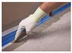
9. Spread on a second layer of the specified MAPEI waterproofing product to completely cover the edges of the tape so they are sandwiched between the two layers of the cementitious mortar
